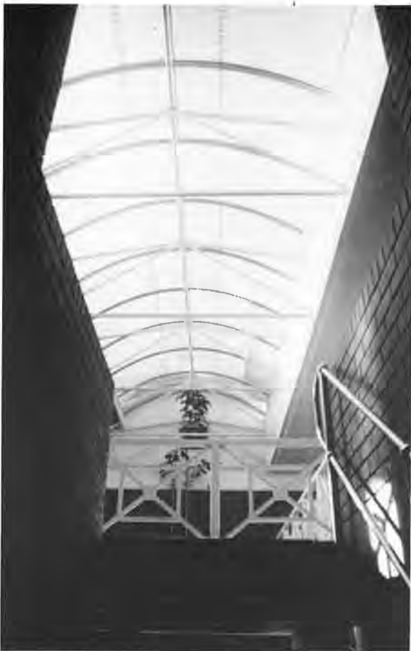
Portion of the roof light at the stair termination.
