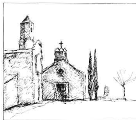
VIEWPOINT I On passing through the covered gateway a view of a small chapel dominates.
