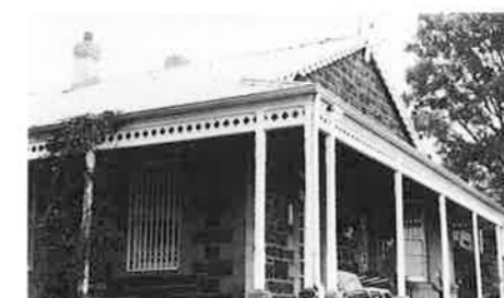
The prototype of the Ladysmith house: the residence of the magistrate, c1890. A core well shielded from the influence of the sun, and a gabled ventilator dormer to release hot air build-up.
