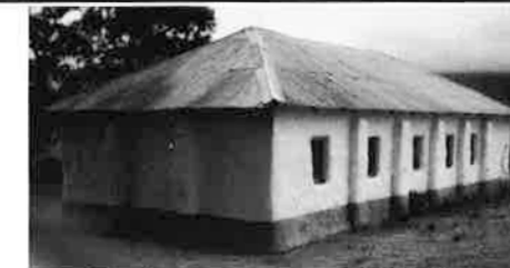
Typical church in the Umzimvubu parish: daubed walls with piers and corrugated iron roof
