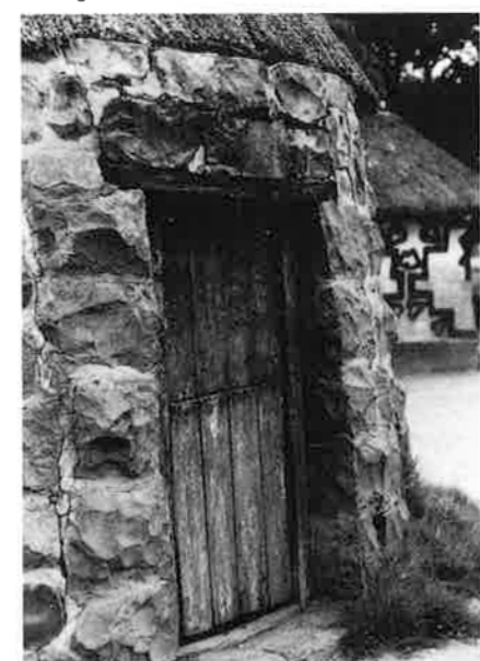
BELOW: Existing rondavel of battered bluestone walling
