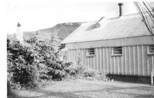
ABOVE: Setting above the Mzimkulwana River. At left, the nature reserve FAR LEFT: East and west gable walls are faced with natural stone LEFT: South wall of asbestos-cement sheeting with fiberglass insulation BELOW: Interior
