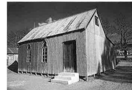
St. Michael and All Angels, Cedarville, a corrugated iron church consecrated in 1915. Painting of roof and new door sponsored by Natal Architectural Heritage Committee
