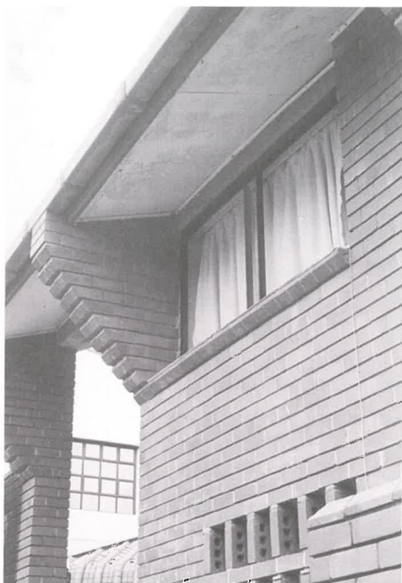
Corbelled plinth headers to the wing wall of a student room.
