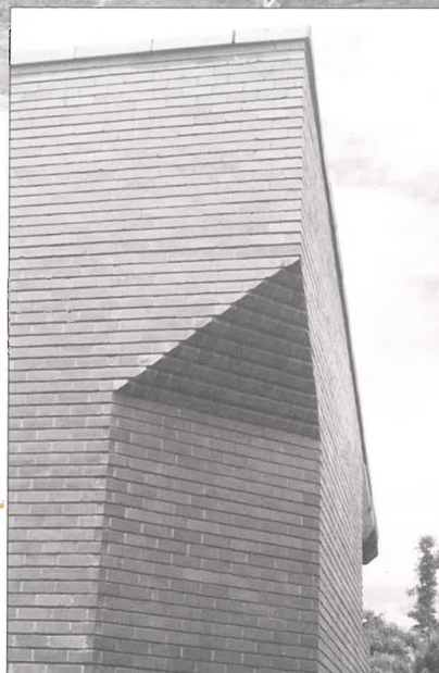
Corbelled plinth headers to the wing wall of a student room.
