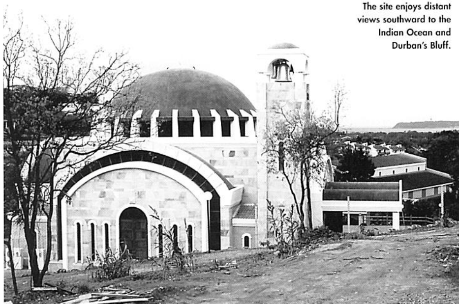
Photograph of the model for the 1988 Design Dissertation. In the realisation, the sides to the dome have become segmented barrel vaults, which butt against the cubical base to the composition, a junction more closely aligned to the precedent, Hagia Sophia, begun circa 532. The bell tower of the dissertation at the entrance has become a campanile, integral with the church. The community centre, foreground left, was built first.
