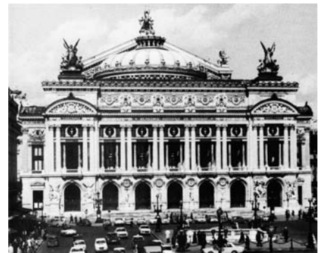
2 Paris Opéra, 1862-75, an example of Beaux-Arts planning which sought the simplest possible circulation into and through a building, and the clear expression of the various functions through separate volumes. Architect Charles Garnier.
