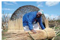
Thatching commences with the affixing of the perimeter mat of ubhaqa grass.
