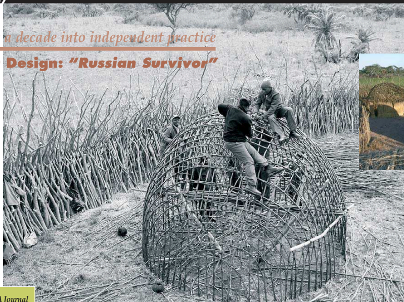
Completing the domical structure formed by arches in two directions on plan. Below left: Saplings bent and tied to form arches from four points of ignition.
