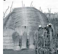
Thatching commences with the affixing of the perimeter mat of ubhaqa grass.
