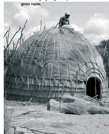
Mist-belt ingongoni grass layered beneath the woven grass ropes.
