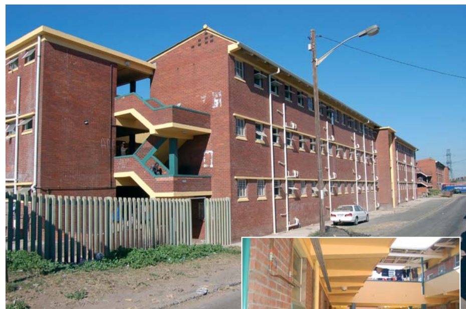
Apartheid legislation set window cills at 1800mm above floor level. Pull strings were added to provide for opening and closing of windows.
