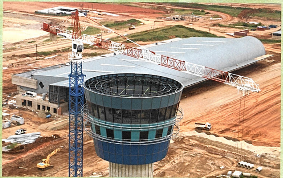
ABOVE: Background—Cargo terminal: NSM Designs; Foreground—Control Tower: Shabangu Architects. Cab module lift completed.
