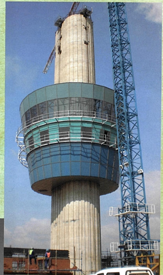
Structural steel 3-D assembly framework of cab.
