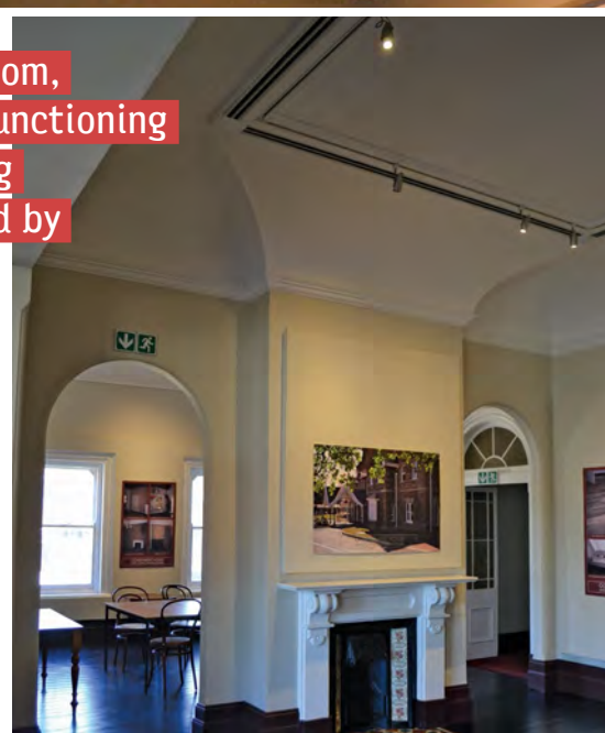
ABOVE: New gallery – air-conditioning diffusers integral with the lighting track. BELOW: New staircase in new stairwell.
