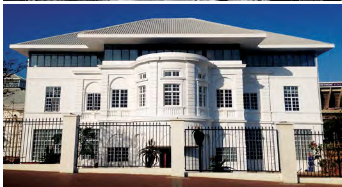
TOP: Aerial view from the 1940s. ABOVE AND RIGHT: In the current rejuvenation, the projection of the lift tower and the conical roof to the bay were disposed of.
