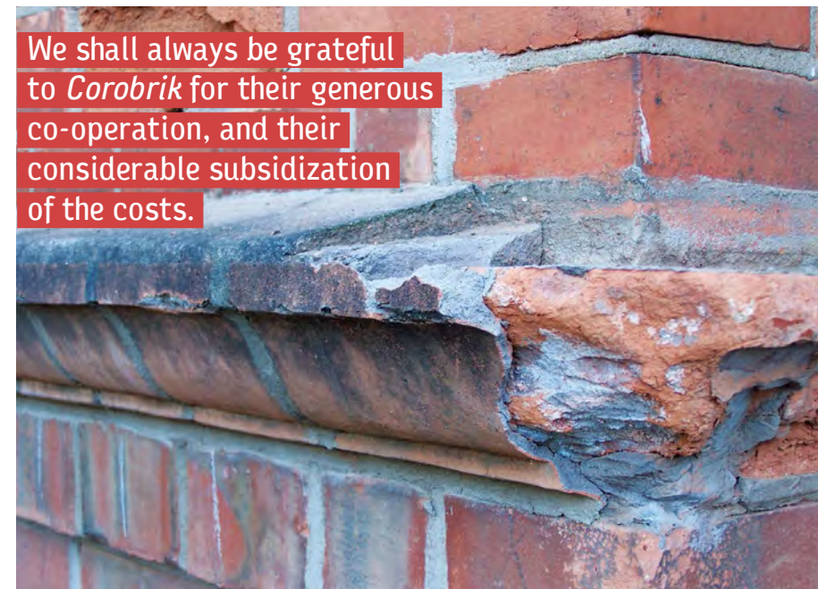
ABOVE: Damaged brick courses which, despite earlier experiments of replacing with mortar and brick dust finish simply had to be replaced. BELOW: Drawings of replacement bricks that were specially manufactured by Corobrik .
