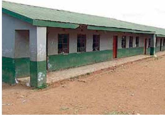
Classrooms before demolition
