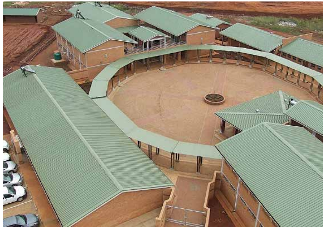
Aerial view of Langa Secondary School
