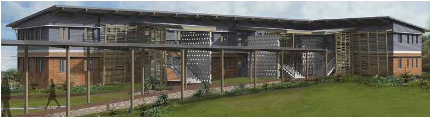
Building 4 seen from the south-west
