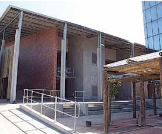
View of the piazza from the east
