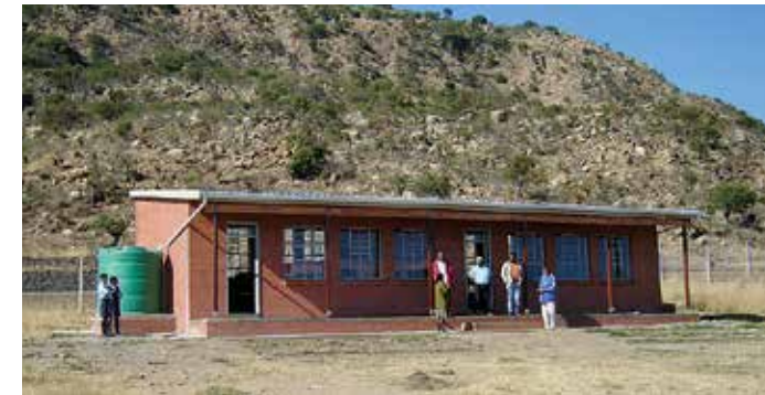
New classroom block at Qhobo
