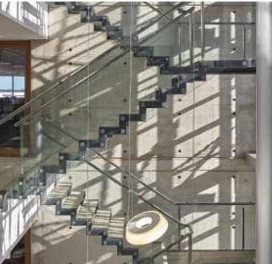
Details of the suspended stair flights.
