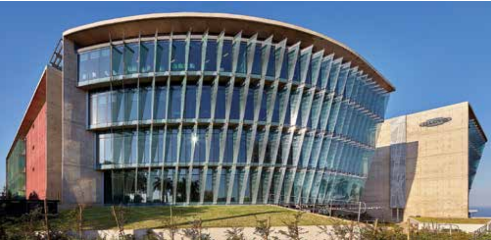
The effect of the inclement sun on Umhlanga Rocks and Kikembe Drives is mitigated by vertical baffles or fins of fritted glass. Editor
