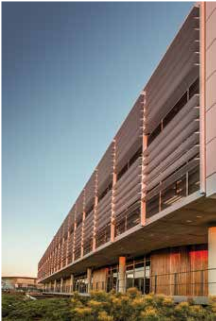
The northern façades, whilst also glazed floor to floor, are protected with a system of deep aerofoil louvres set off the façades and angled to cut out solar gain throughout the year whilst affording occupants views inland.
