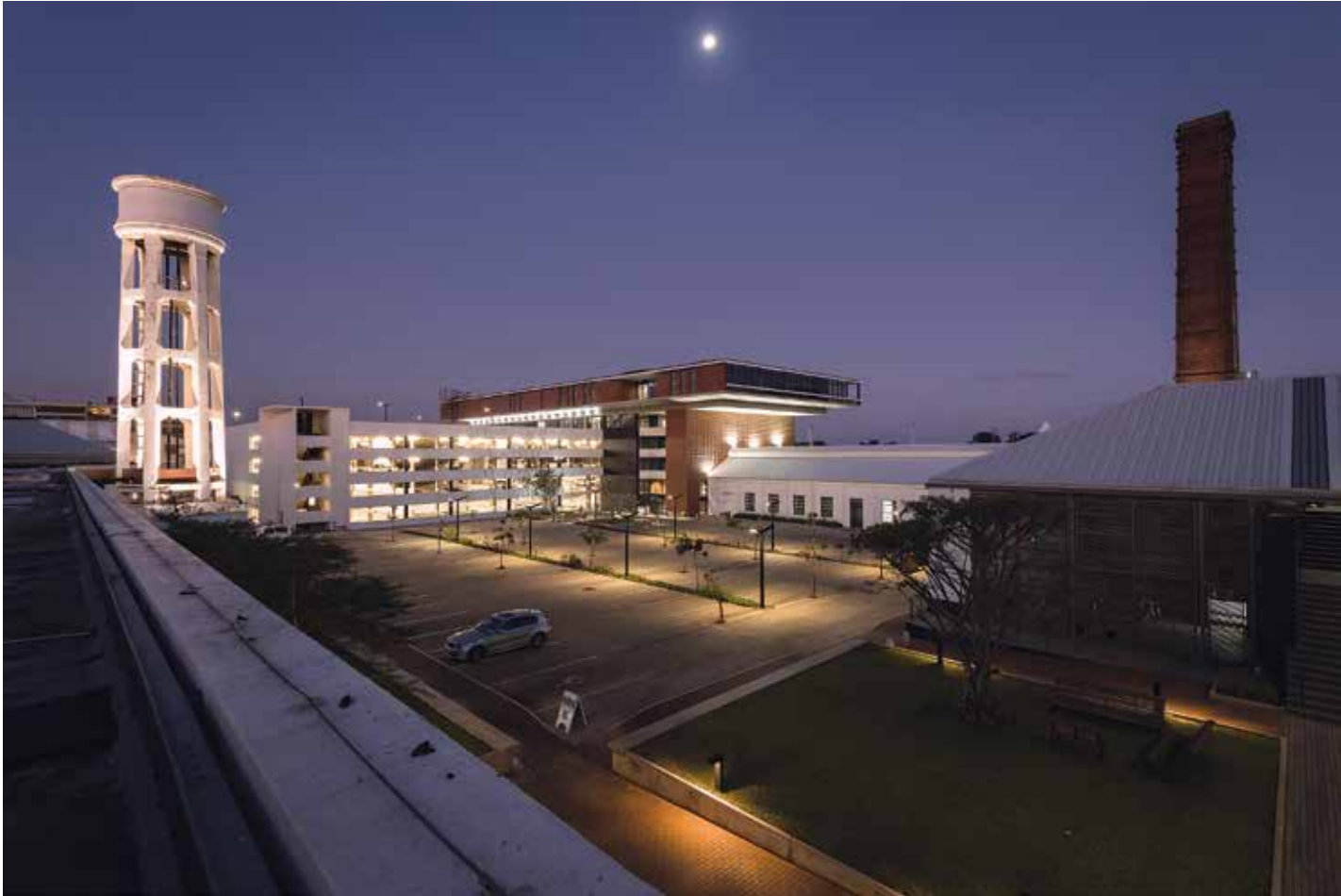
Evening shot looking north-east with JT Ross House in the context of the historical Lion Match Park. The 20m cantilever was prompted by the client's requirement for 2 500 sqm office space on one floor facing the Indian Ocean. This enables the spatial and view requirements without in any way infringing on the heritage protected abutting building.
