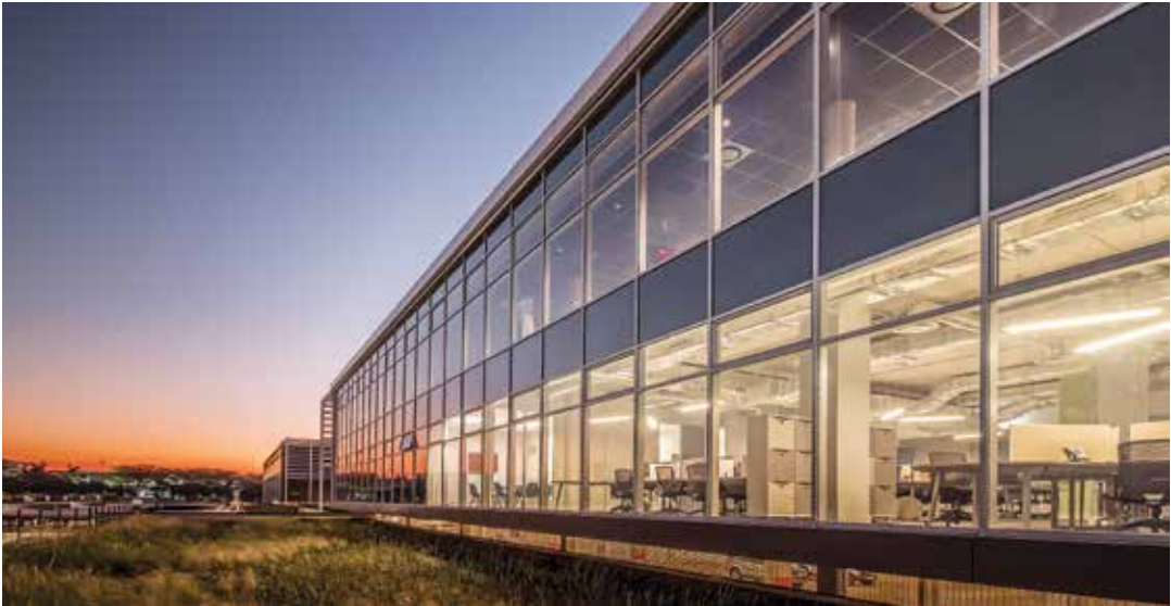
The southern façades are fully glazed to take advantage of the expansive city and ocean views. All the blocks float above the indigenous landscaped roof slab that covers an extensive basement parking level.
