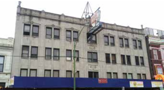
Former Diplomat Hotel before the intervention. The existing windows had single-pane glazing, which was not energy-efficient. Exterior masonry was damaged and spalling caused by the freeze-thaw cycle in cold climates.
